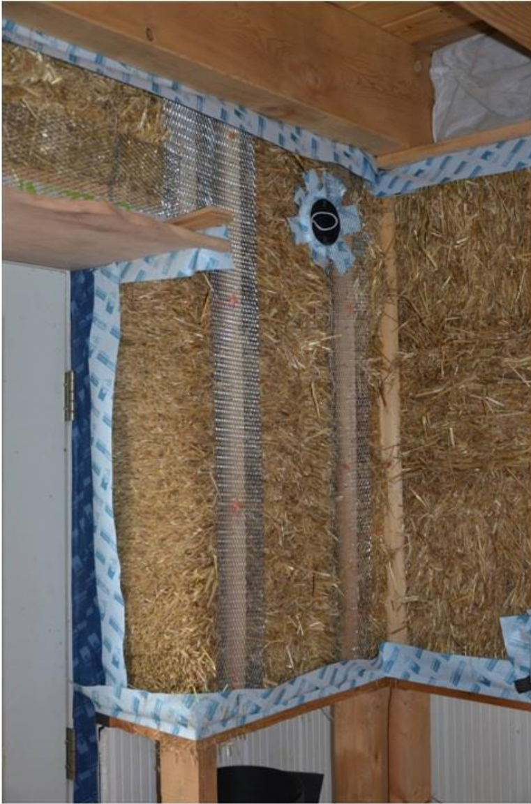
New Frameworks Construction
