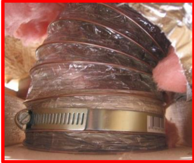
Connection in place but not sealed.
