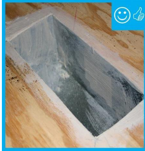
Courtesy of the Department of Energy's Building America Solution Center ( http://bas.energy.gov )
