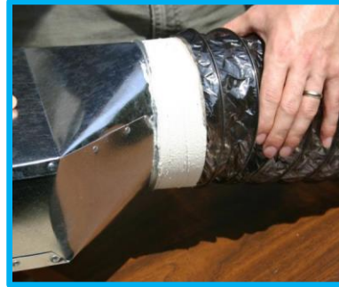
Mechanically fastened and sealed.
